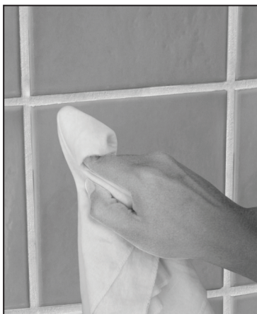
Cleaning using lint-free cloth
