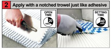
Dampen surface before application. Spread ABC 2 in 1 mortar with a notched trowel & position mosaic tiles immediately within 20 minutes open time. Press mosaic tiles with a rubber float to ensure good bonding & 100% mortar coverage. Use tile spacers for proper alignment & remember to carefully remove them before adhesive sets. Let tiles set for about 40 minutes. Do random checks to make sure all tile pieces are level & all tile sheets are properly adhered.
