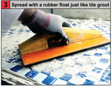
Start grouting with a rubber float by spreading 2 in 1 mortar diagonally across the tile joints making sure all joints are uniformly filled. Wait for 5 minutes & carefully remove excess mortar with a damp sponge using diagonal strokes. Remove haze with a clean, damp & lint-free cloth. Don't allow excess mortar to harden on tiles since it will be difficult to remove later on.
