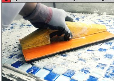
Start grouting with a rubber float by spreading 2 in 1 mortar diagonally across the tile joints making sure all joints are uniformly filled. Wait for 5 minutes & carefully remove excess mortar with a damp sponge using diagonal strokes. Remove haze with a clean, damp & lint-free cloth. Don't allow excess mortar to harden on tiles since it will be difficult to remove later on.
