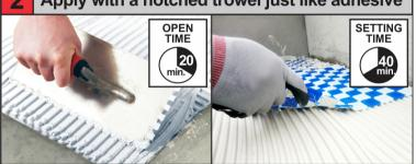
Dampen surface before application. Spread ABC 2 in 1 mortar with a notched trowel & position mosaic tiles immediately within 20 minutes open time. Press mosaic tiles with a rubber float to ensure good bonding & 100% mortar coverage. Use tile spacers for proper alignment & remember to carefully remove them before adhesive sets. Let tiles set for about 40 minutes. Do random checks to make sure all tile pieces are level & all tile sheets are properly adhered.
