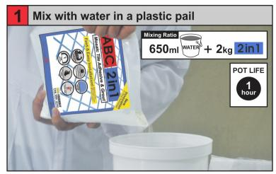
Pour clean water into a container & add ABC 2 in 1 powder. Stir to attain a lump-free, creamy consistency. Use immediately after mixing and strictly observe 1 hour pot life.
